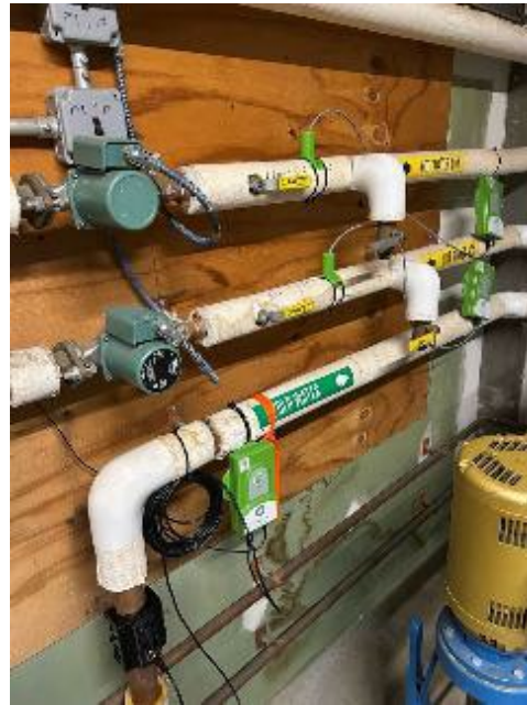
Figures 2 and 3. Evolution Temperature Sensors on domestic hot water (DHW) piping.
