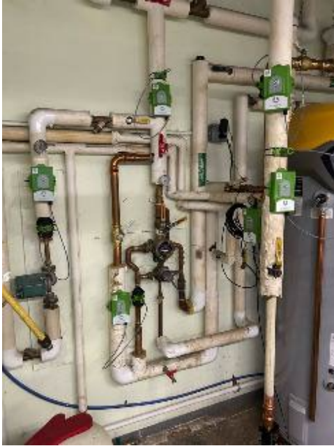
Figures 2 and 3. Evolution Temperature Sensors on domestic hot water (DHW) piping.
